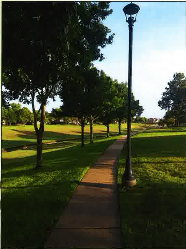
Trail Lighting LED Lamp Post
