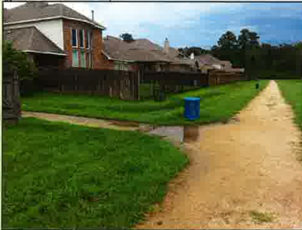
Low depressed areas holding water at trailhead connections.
