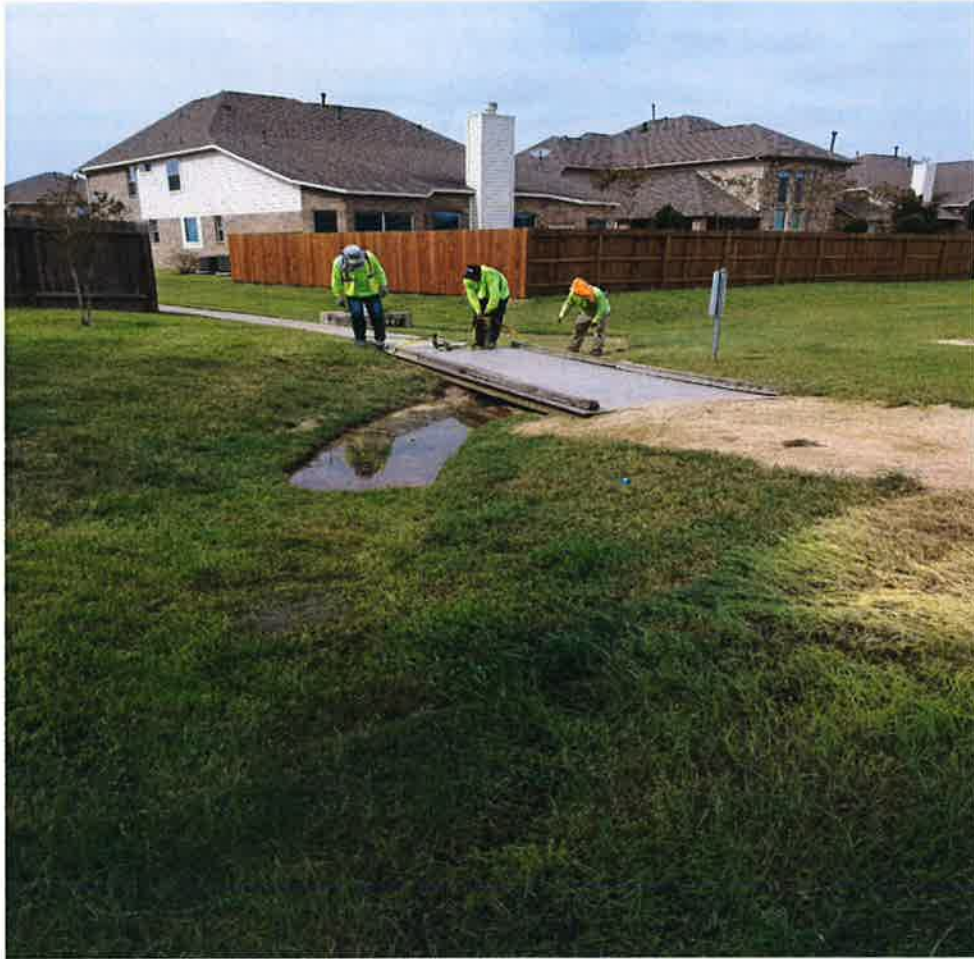
Foot bridge is re-installed across the back slope swale ditch
