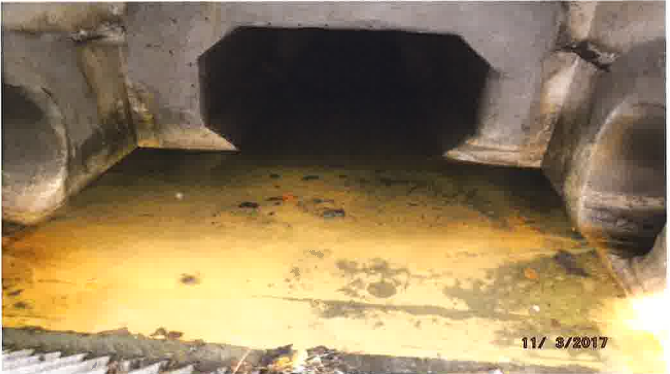
View inside with storm drainage pipe connections.
