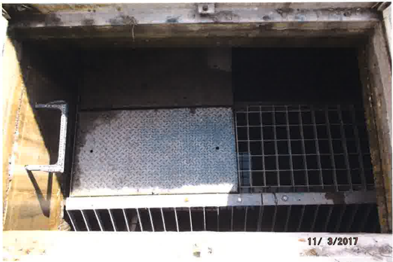
View upon opening the doors.
